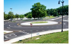
Roundabouts are designed to improve safety and traffic flow by reducing conflict points and lowering vehicle speeds. Unlike traditional intersections, they virtually eliminate the potential for highspeed, right-angle, and head-on collisions. They types most likely to result in serious injuries or fatalities (FHWA, n.d).
